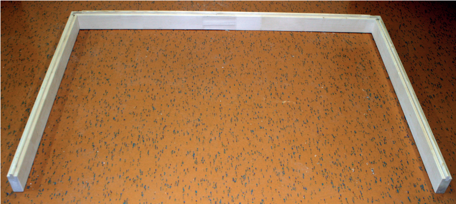
Fig. 1: Placing the three floor frame elements
