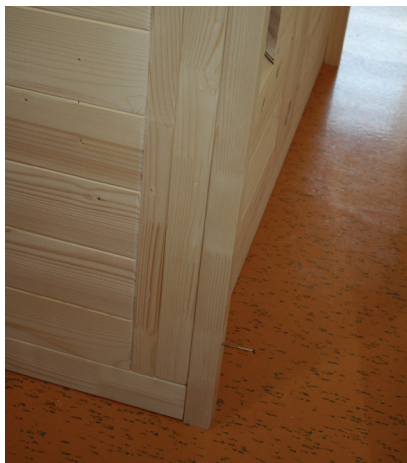
Fig. 52: Installation of the spacer strips of the rear wall
