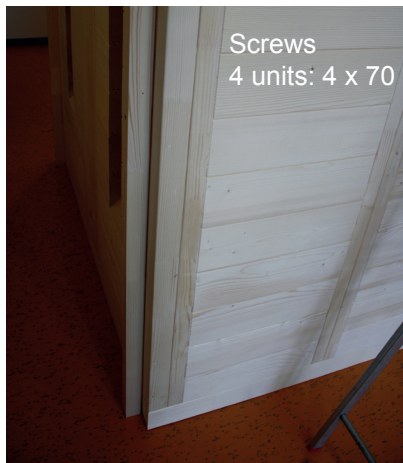
Fig. 52: Installation of the spacer strips of the rear wall
