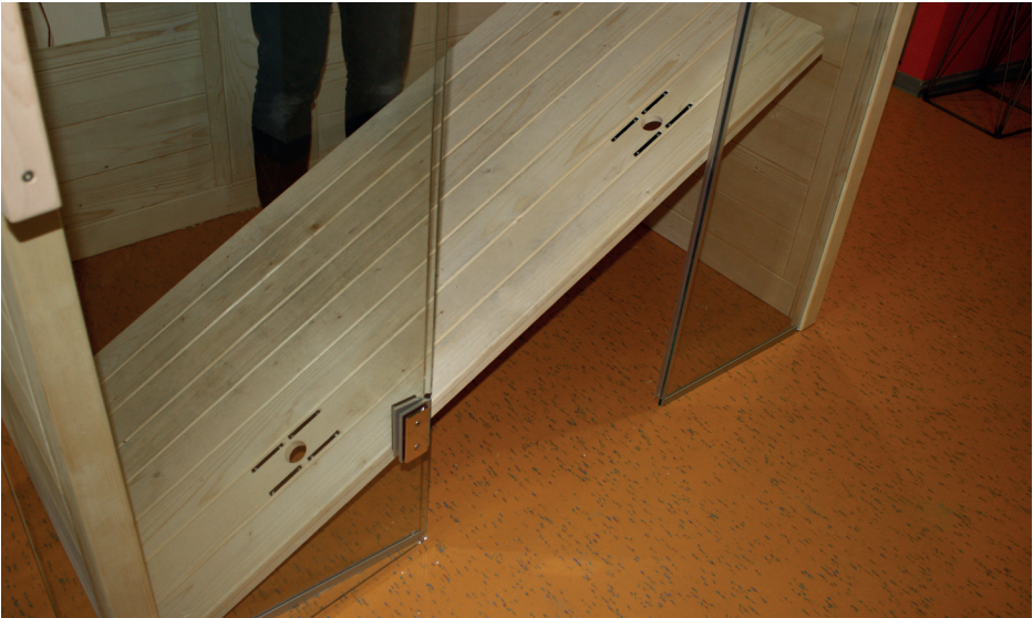
Fig. 28: Put the cabin floor in place
