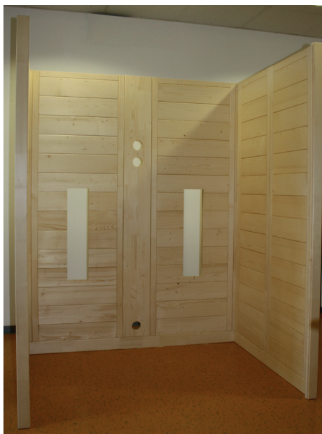
Fig. 10: Installed wall elements
