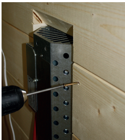
Fig. 42: Installing the rear radiator blind
