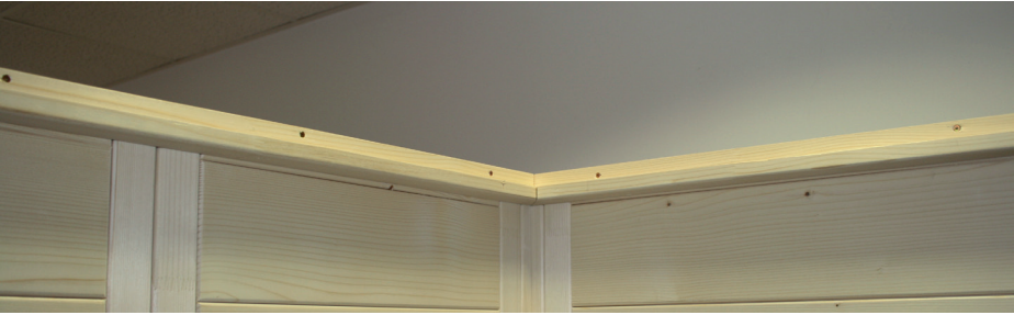
Fig. 17: Installing the roof element in the back with the fan cut-out
