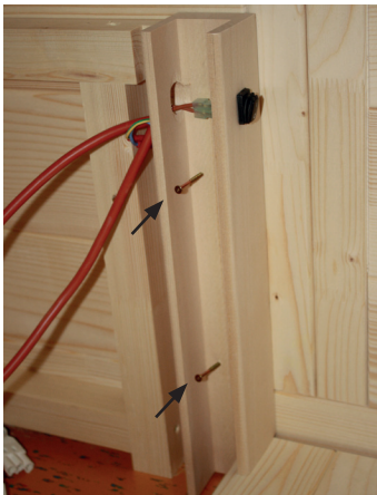
Fig. 33: Installation of the U-strips for the thermal plates
