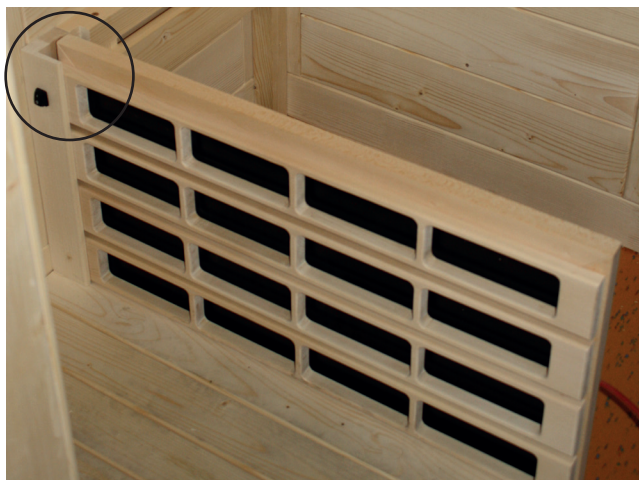
Fig. 34: Installation of the IR thermal plate VitaMy 164
