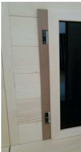
Fig. 53: Installing the backrests of the bench
