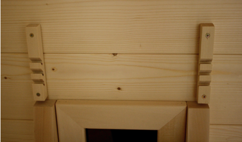
Fig. 54: Installation of the headrests
