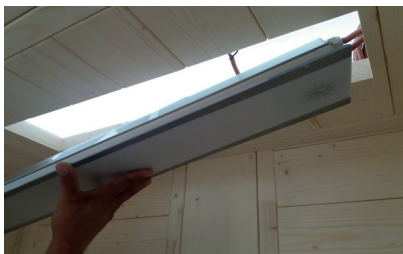
Fig. 50: Installing the colour light
