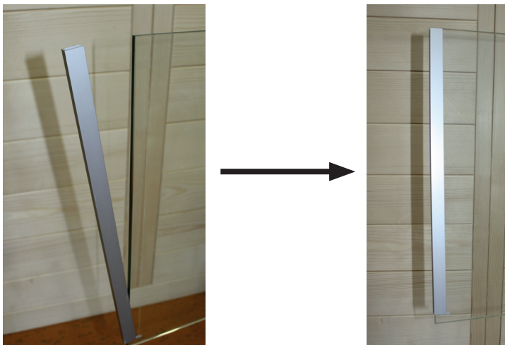
Fig. 11: Attach the U-profiles to the glass plates
