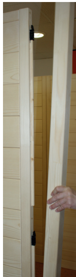
Fig. 9: Installation of the two front corner posts with a groove for glass
