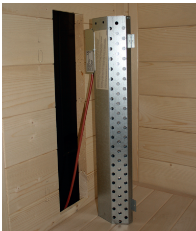
Fig. 41: Install the rear radiator (infrared radiator ECO 350)
