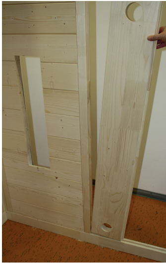
Fig. 6: Install the electrical element in place
