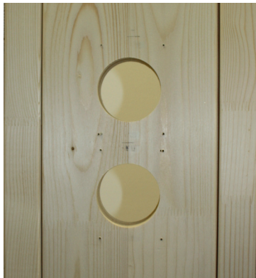
Fig. 46: Installing the control panel
