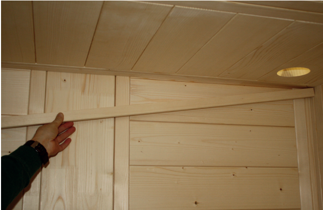
Fig. 37: Installation of the LED cover strip
