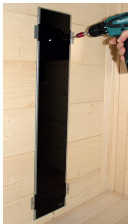
Fig. 41: Install the rear radiator (infrared radiator ECO 350)
