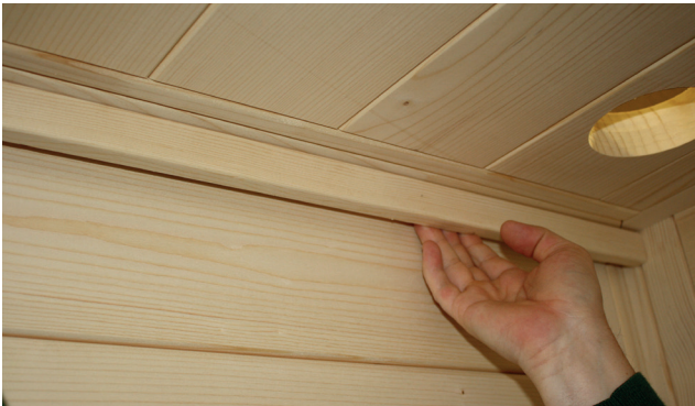
Fig. 38: Glueing the LED strips in place
