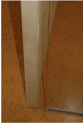
Fig. 12: Inserting the glass sheet in the groove of the corner post
